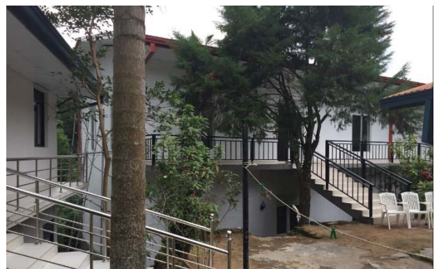
Training Institute Building in Kadugannawa, Sri Lanka to which the UK Community donated through the International Collaboration Fund in August 2013
