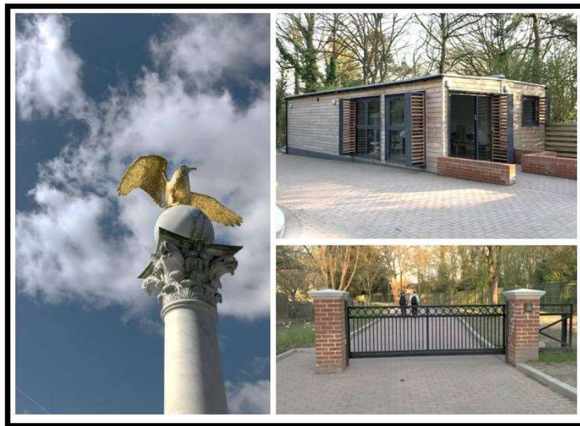
Restoration and new construction work at the Guardian's Resting Place is now almost complete.
