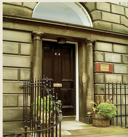
The Edinburgh Bahá'í Centre has undergone renovations to make it a suitable venue for intensive training events, youth weekends and other gatherings.
